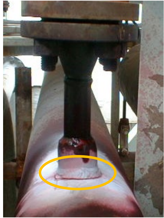
FIV failure of a branch connection
