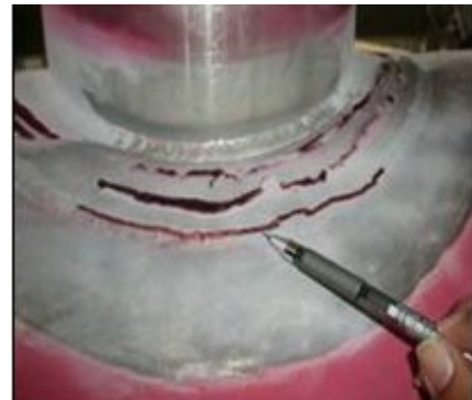
AIV failure at a reinforcement pad weld
